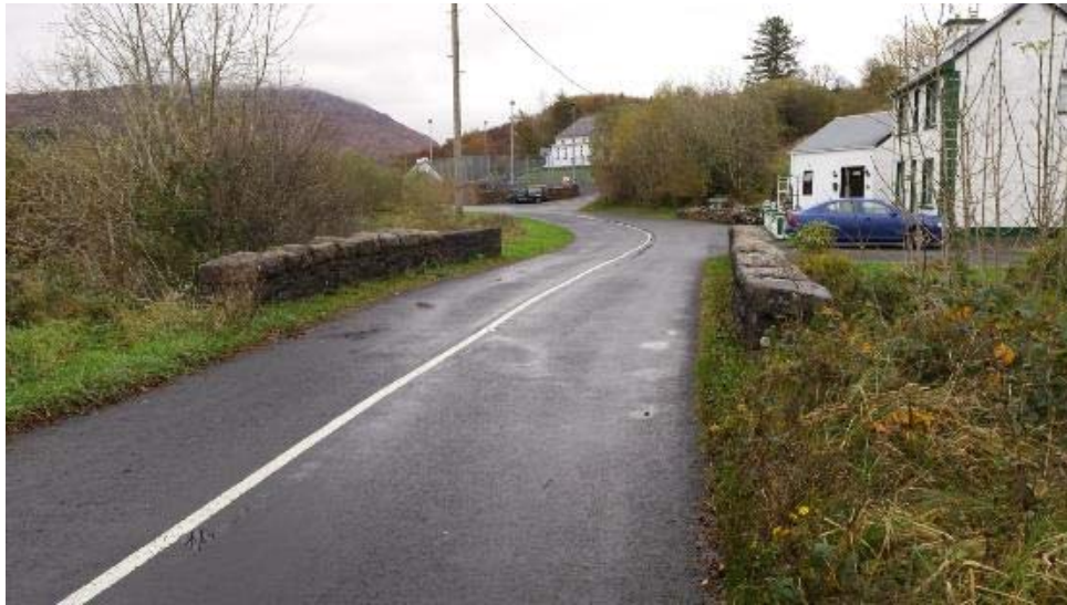
Plate 1-59: NIAH Ref. 40909424 Road Bridge at Cullionboy and Keadew Upper Tds.
