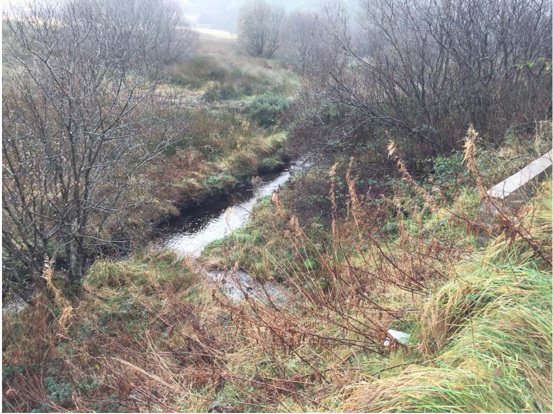
Plate 1-56: Section of proposed underground cable route in the vicinity of culvert where it exits bog, south of N15, looking south
