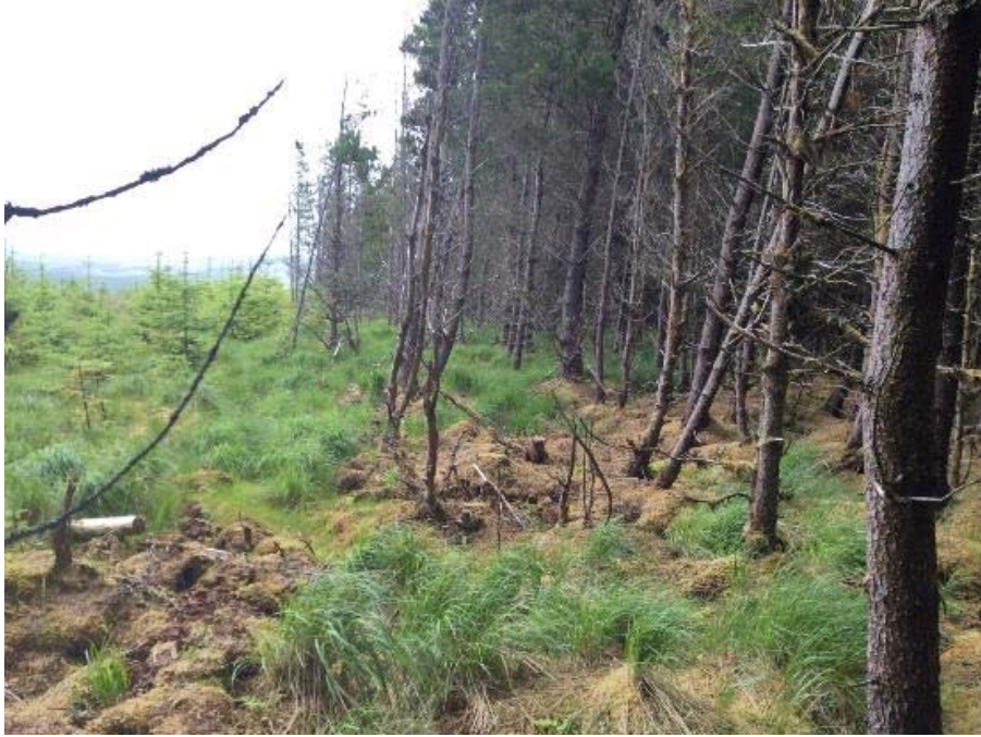
Plate 1-31: Proposed turbine base at junction between mature and young forestry looking north
