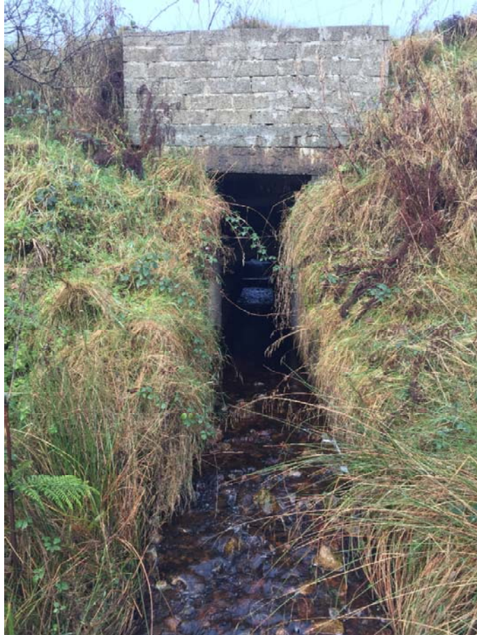
Plate 1-55: Culverted stream at ITM E604244, N 887465 south of the N15
