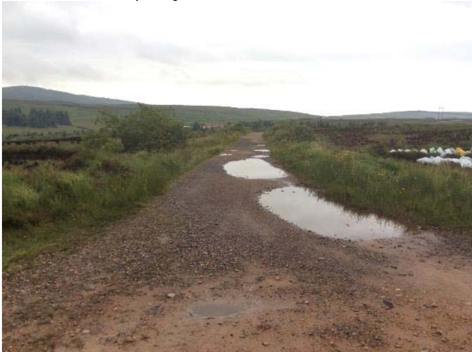
Plate 1-52: Continuation of grid connection route looking north towards quarry
